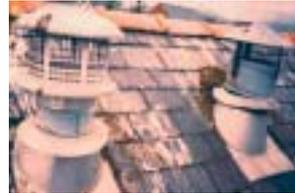
Gulls could nest on flues and block them possibly resulting in accumulation of noxious gases inside buildings
